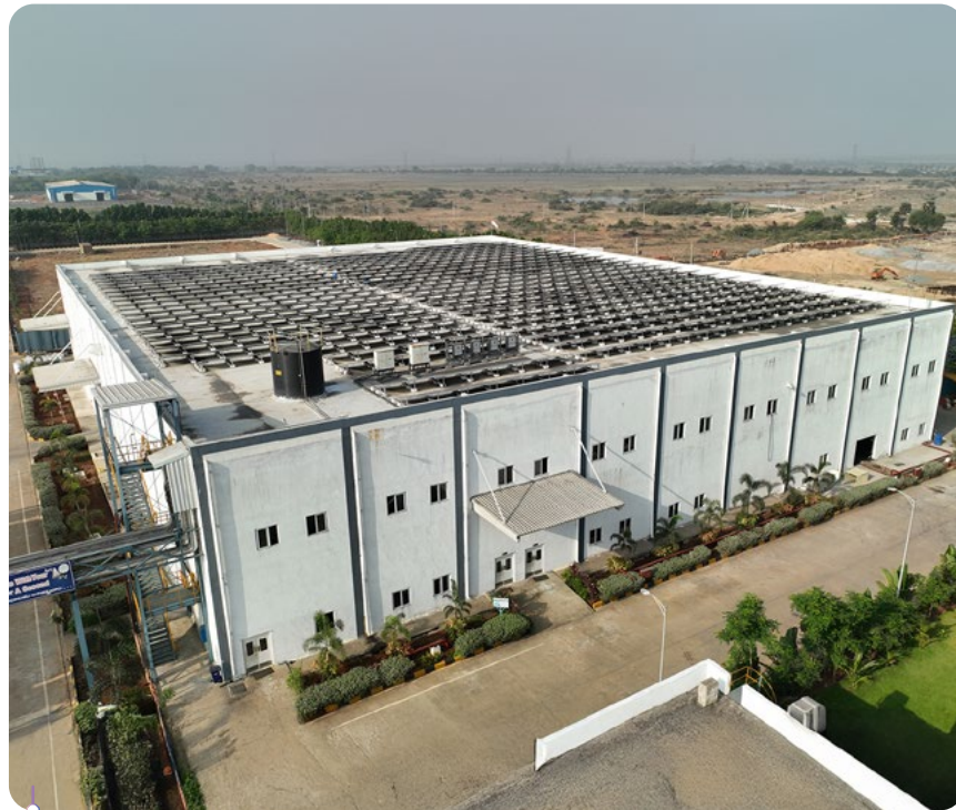
Agro Formulation facility, Attivaram, Andhra Pradesh
